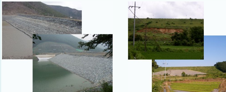
Reinstallation of rip-rap (YCdDam, AGDam)
