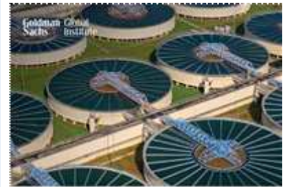
Securing and Financing the Future of Water
